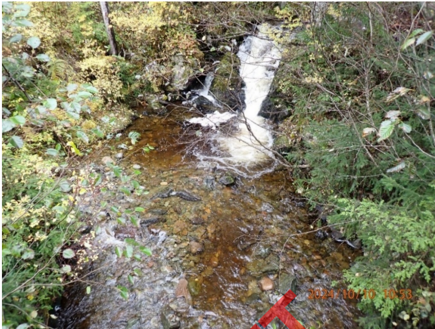
Figure 9: Looking upstream from the existing bridge across Cascade Creek. A scour hole has developed directly downstream of a series of cascades approximately 25 feet upstream of the existing bridge.
