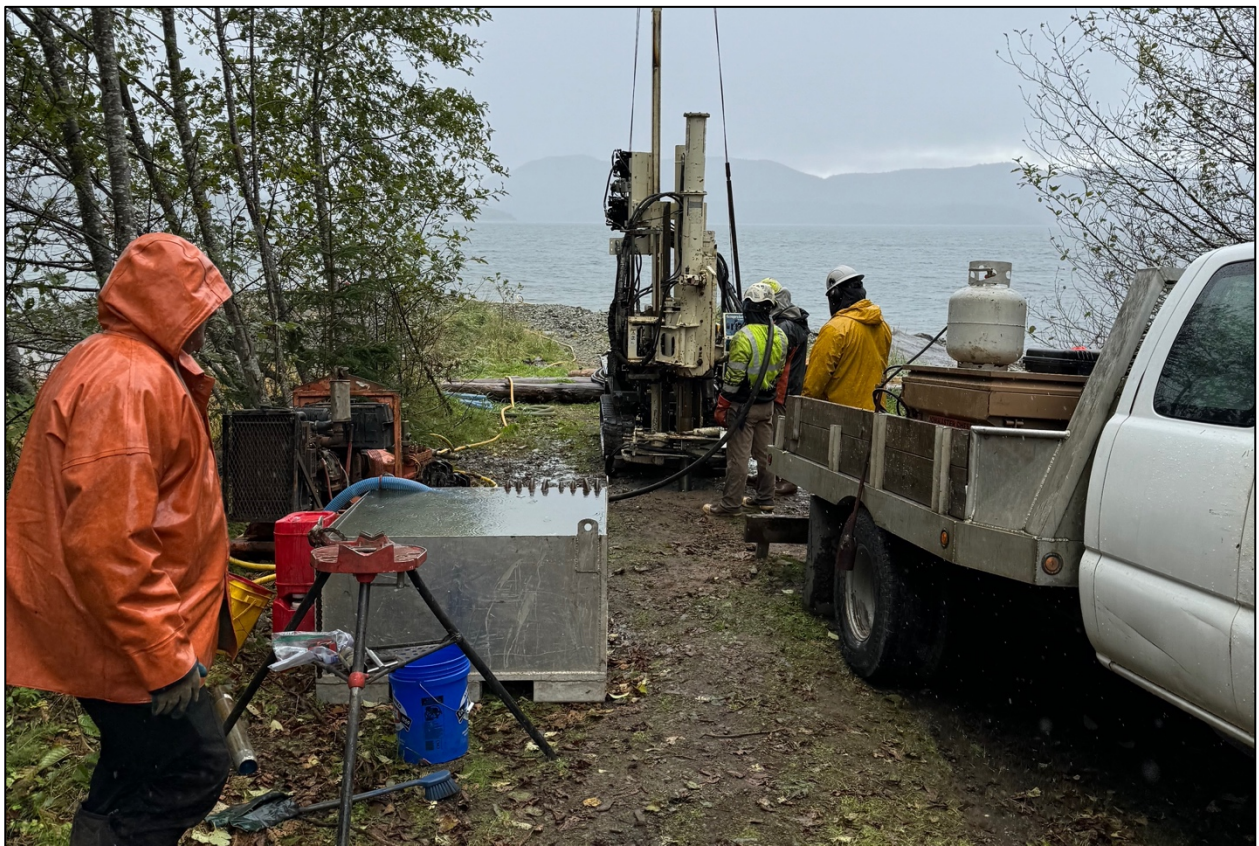
Figure 10. Borehole 21, showing the tracked drill rig utilized for all boreholes.
