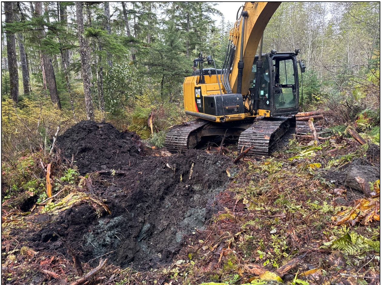
Figure 9. Typical test pit.
